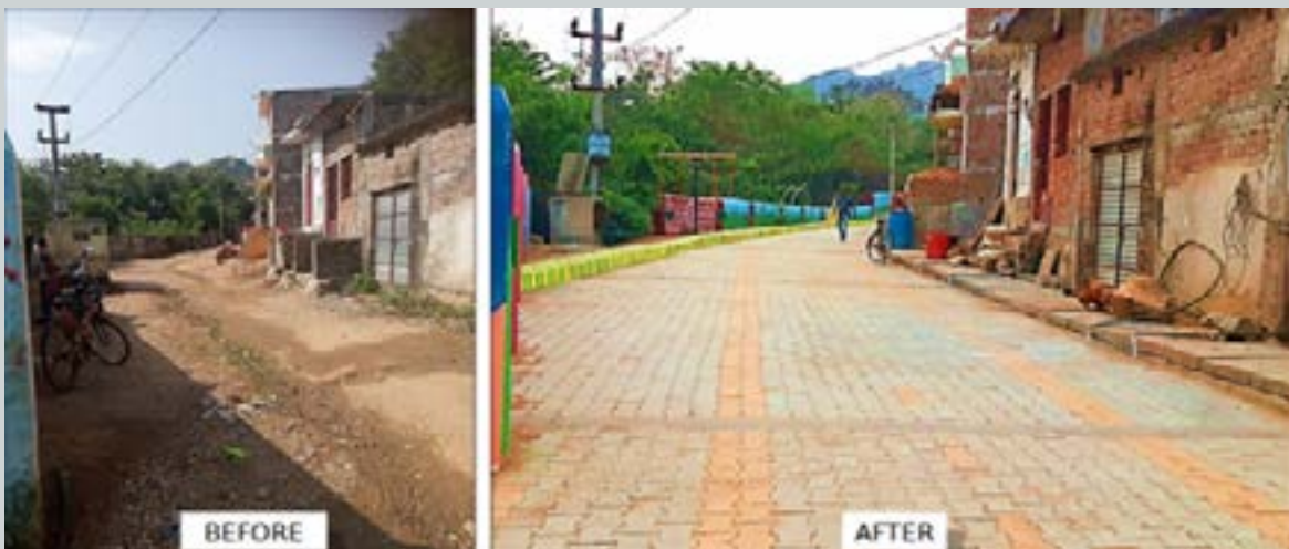
Paver blocks laid for road development in slums of Hinjilicut
